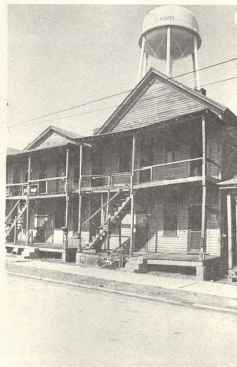
Cairo is number one in Illinois in substandard housing, in the top three in poverty incidence.
